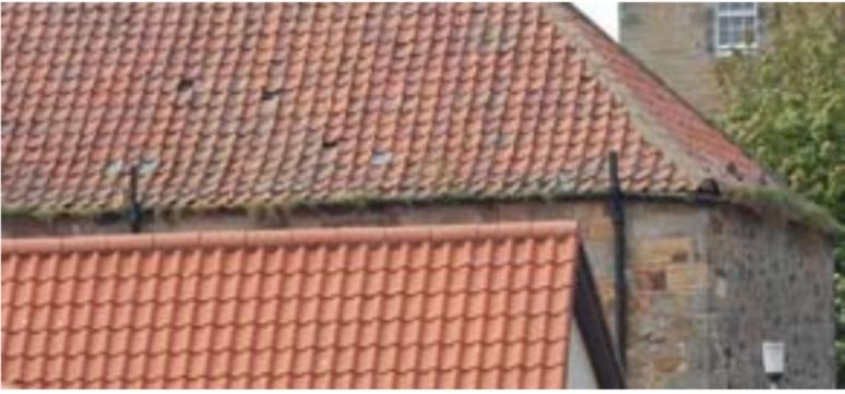
*pantiles should be reused where possible - new tiles can completely change the appearance of a building*
