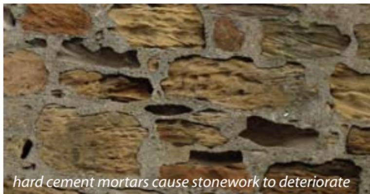
*hard cement mortars cause stonework to deteriorate*
